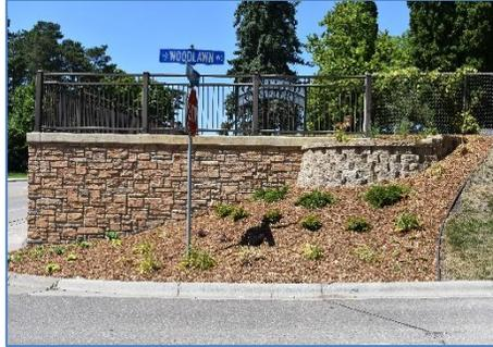
Phase II included removing plantings at the corner of Minnetonka Boulevard and Woodland Avenue. Plantings that could be transplanted to another area were saved. A block retaining wall was added to the slope to facilitate drainage. New low maintenance and low water perennials including grasses, ground cover junipers and several shrubs were planted to enhance the corner. Woodchips were applied to help keep the weeds at bay.
